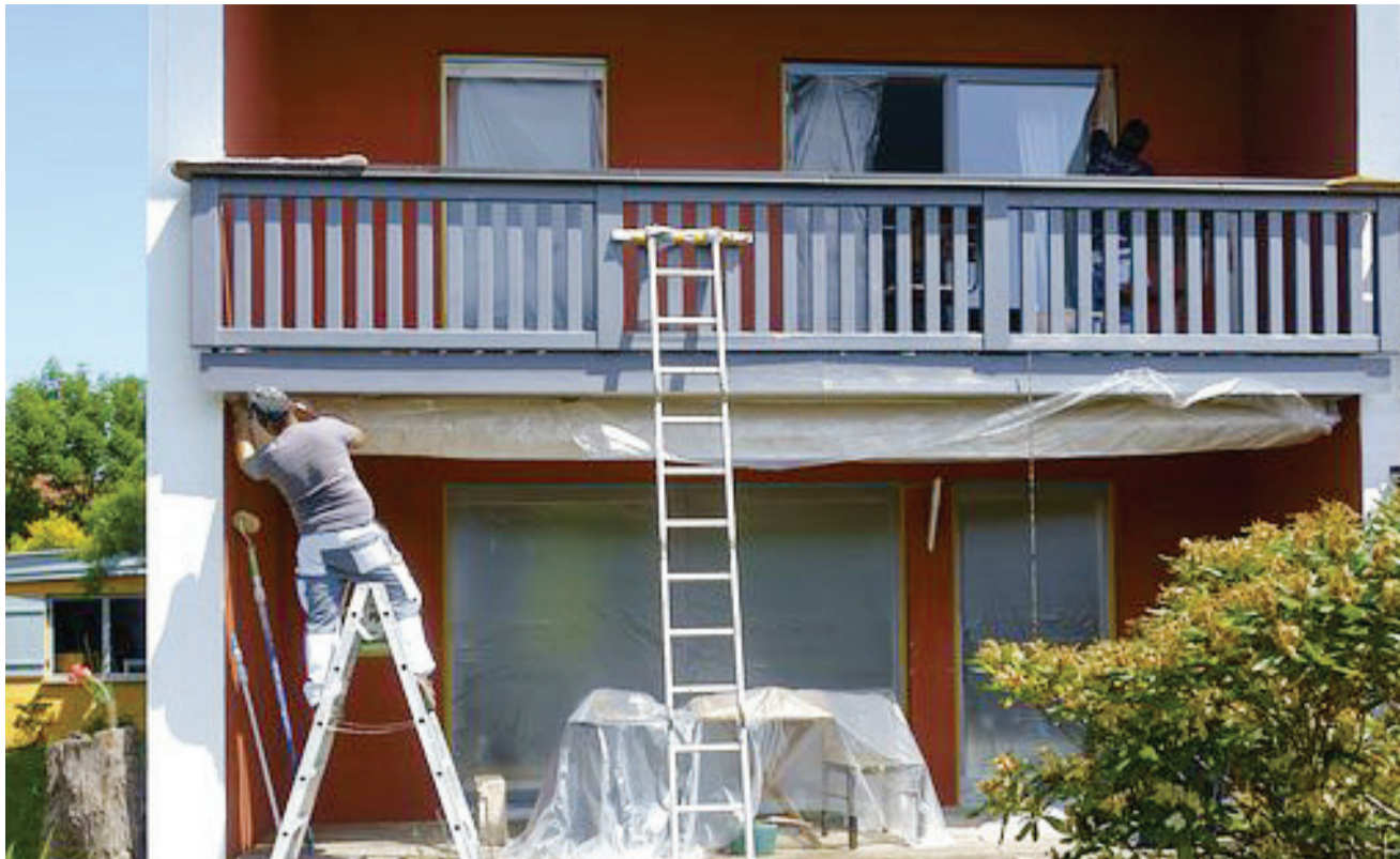
The painting of a building underway.
